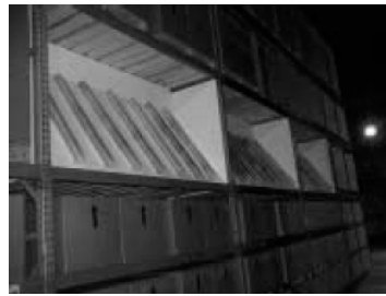
● 12.7.2 Sprinkler Design Criteria for Storage & Display of Class I - IV Commodities, Cartoned Non-Expanded Group A Plastics & Non-Expanded Exposed Group A Plastics in Retail Stores.
